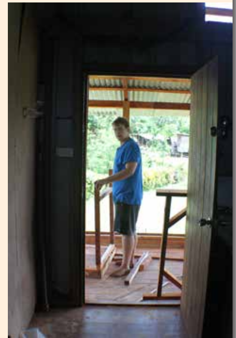
Noah framing deck railing in Papua New Guinea.
