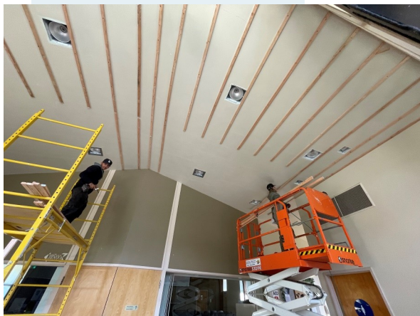
Prepping for the new foyer ceiling
