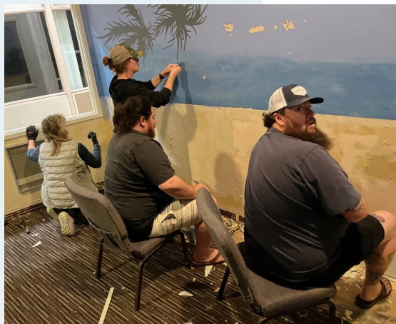
Taking down the cry room
