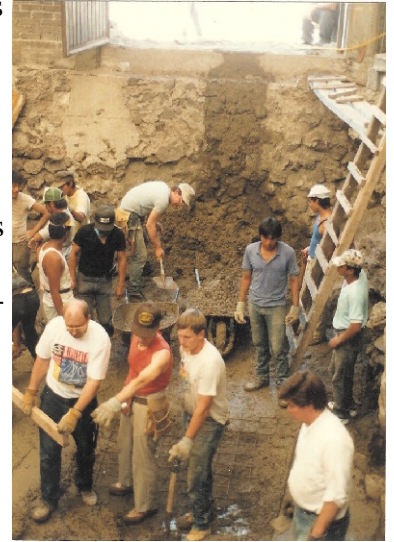
Mexico Mission Trip Construction
