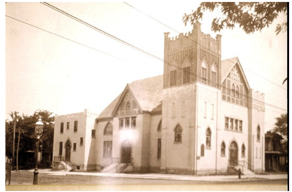
1908 First Free Church at 12th Avenue and 7th Street
