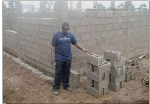
In-Country Director, Pastor George Mbuswe, visiting the building site in Lysoka
