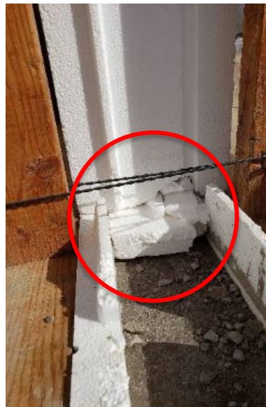
CUT A 1" WIDE 'SEAT' IN THE BLOCK TO ALLOW THE 2X8 FORM TO SIT. THIS FORM IS TEMPORARY AND WILL BE REMOVED ONCE THE CONCRETE CURES.
