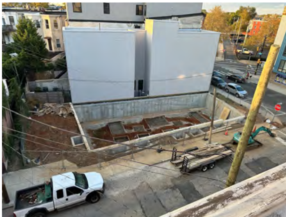
(above) View of new construction from the Kieselowsky's roof.
